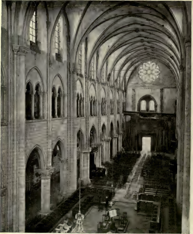
NAVE, LOOKING WEST Church, St. Leu d'Esserent
